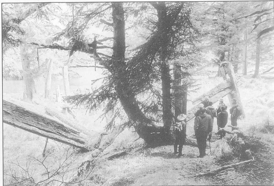
Ninstints corner beams.
